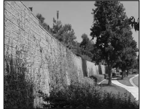
Coherent Gravity Wall
