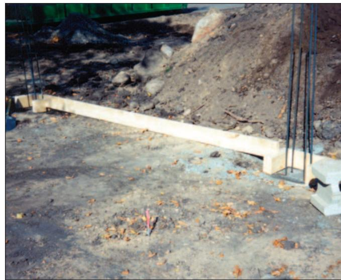
Figure 1: AB Fence Pile Layout Jig
